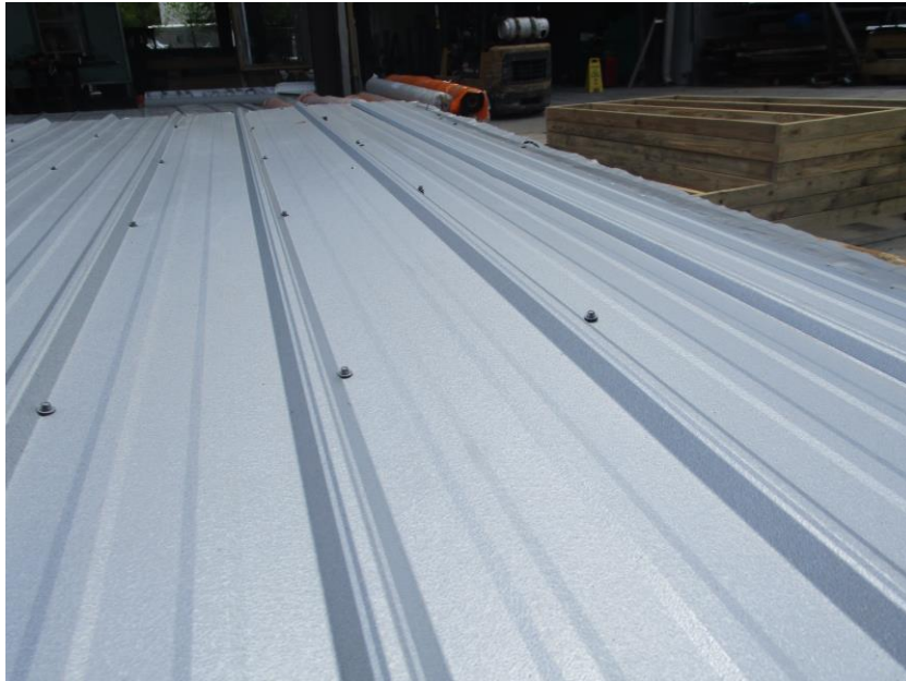
Specimen No. 1 After Testing
